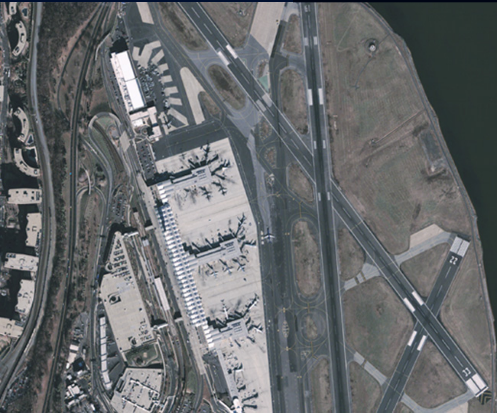
Quick-Bird 衛星影像(DC Airport)
